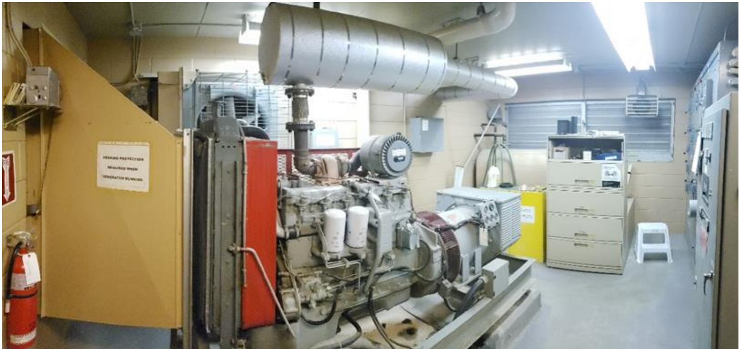
Existing 125 kW Water Street SPS Generator
