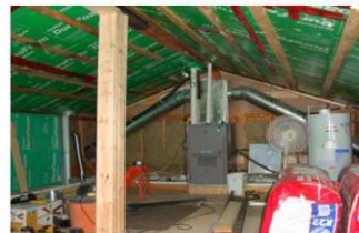
ATTIC FLOOR JOISTS 2"x8" Joist 16" O.C. with solid bridging and 5/8" subfloor
